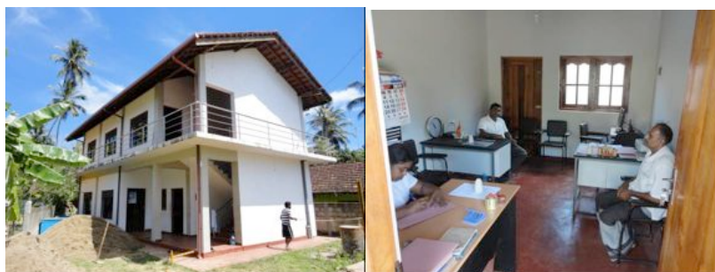
Fig. 4 Kudawella community center where to setup Operation Center Node 2
